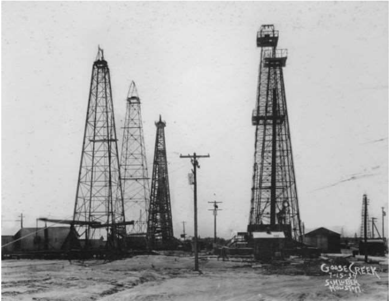
Image 20. This 1934 photograph shows five types of derricks. From left is an early structural steel derrick, a derrick made from tubular steel, a wood derrick and a modern structural steel derrick with a “crow’s nest” on top and another derrick with a crow’s nest and a “fourble board” midway up the derrick. Houston Public Library
