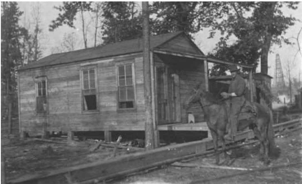
Image 14. So-called “shotgun houses” were popular in the oil field because they were more comfortable than tents. They were delivered by barge and could be easily assembled and moved from place to place as needed. Baytown History Museum.
